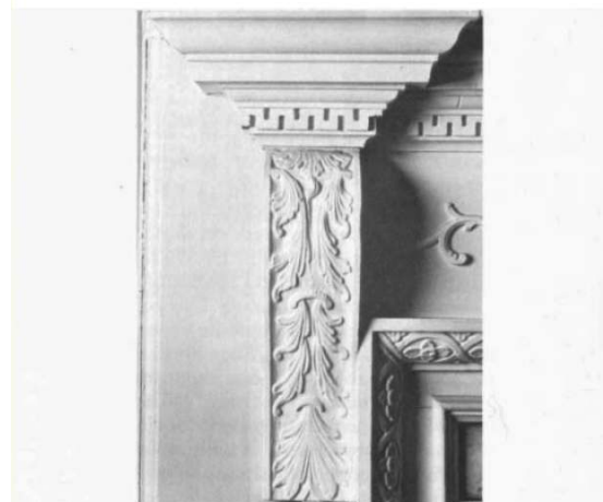
Figure 36. One of the shelf consoles of the chimney piece in the first floor northwest room of the Brice house, carving attributed to William Bampton. MESDA research file S-11401.
